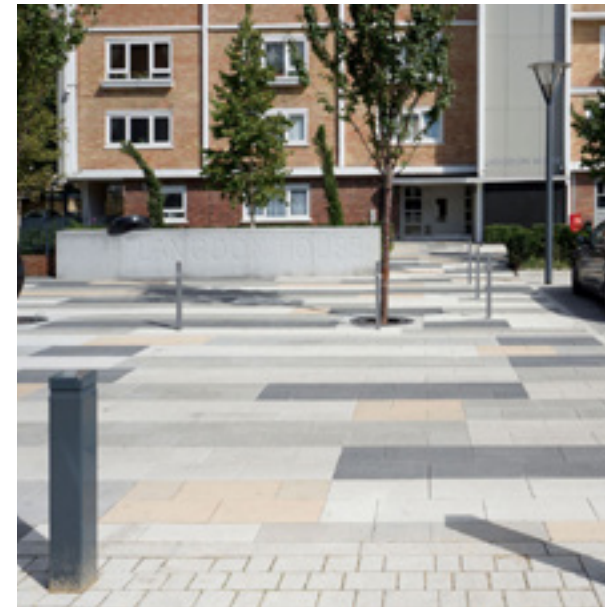
Crossing material prioritises pedestrians at raised table junctions
